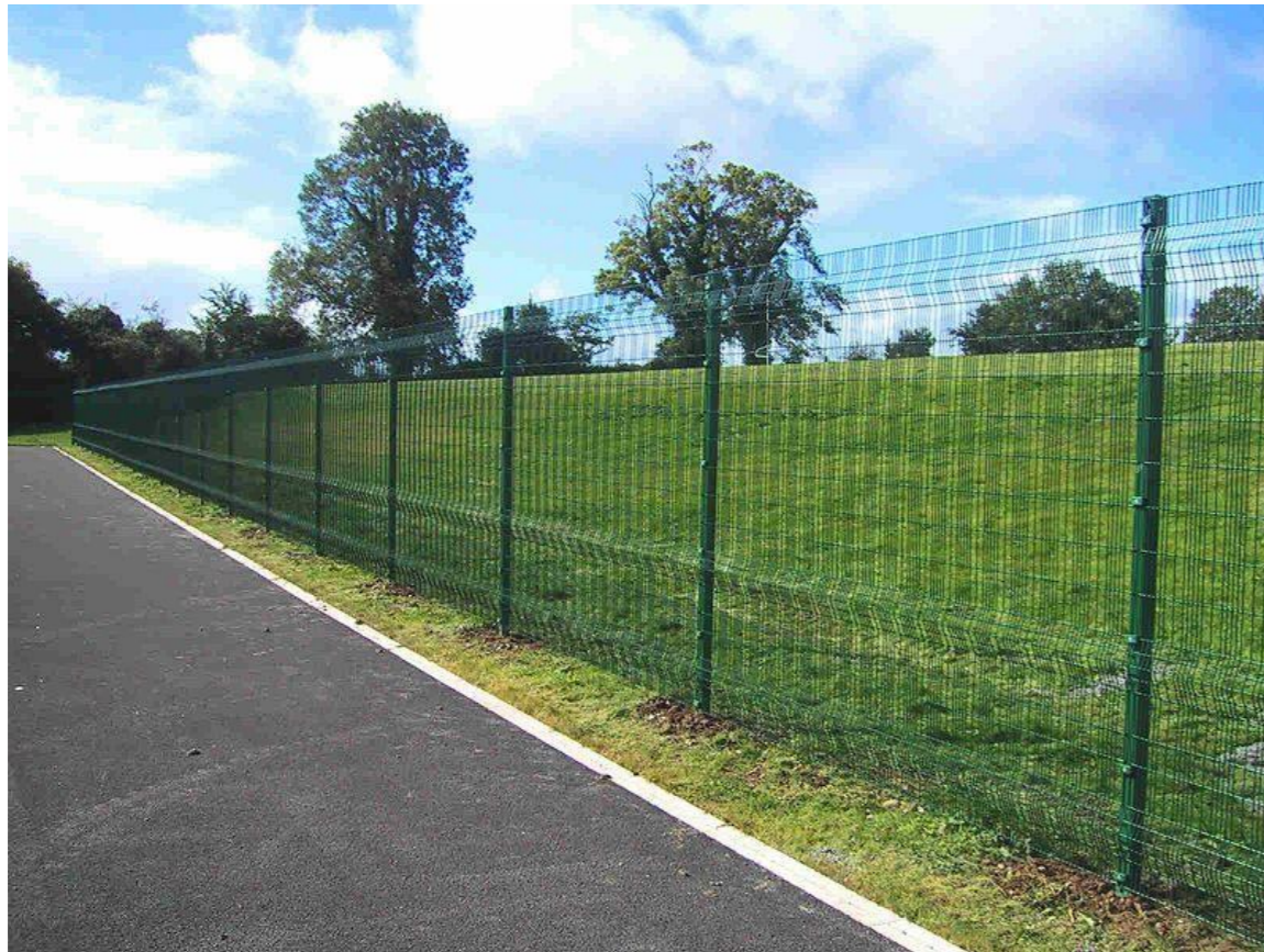
Fig 34. Typical boundary security fencing.
